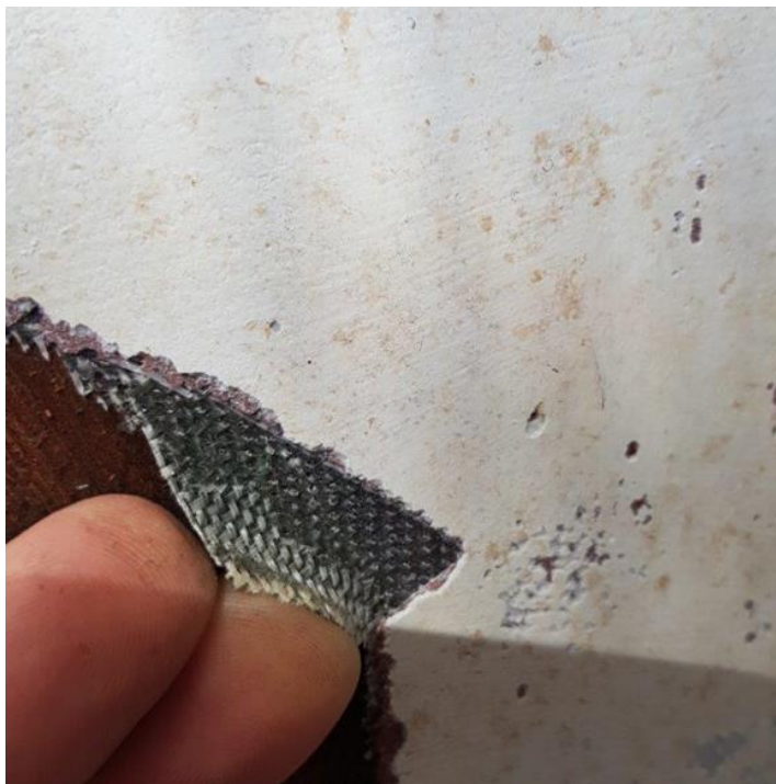
The fiberglass coat is discovered
